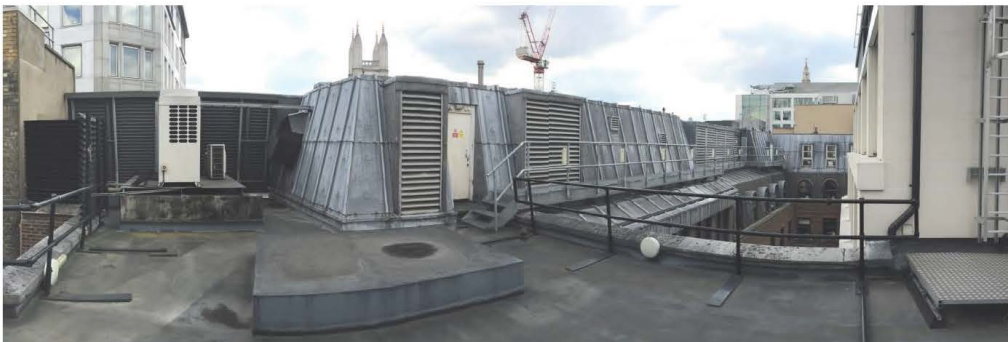
Panoramic views of existing roof & plant enclosures
