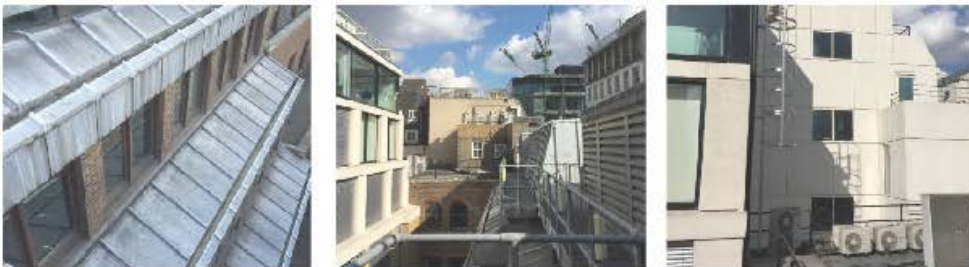
Existing stepped Façade, Existing plant enclosures and neighbouring properties
