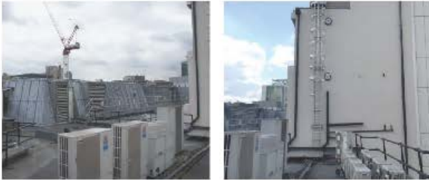
Existing rooftop and means of escape
