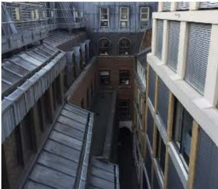
West along Well Court
